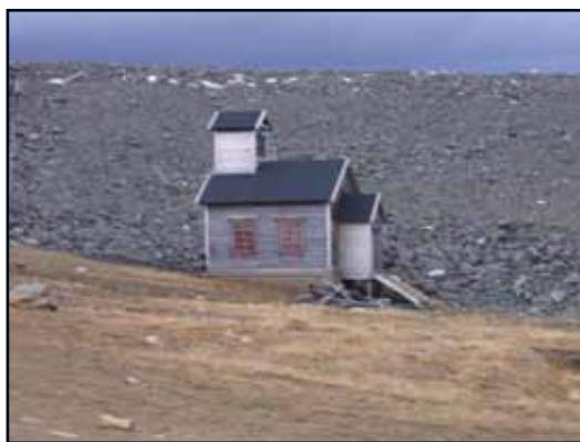
Trafo, Killingdal gruver, Holtålen
